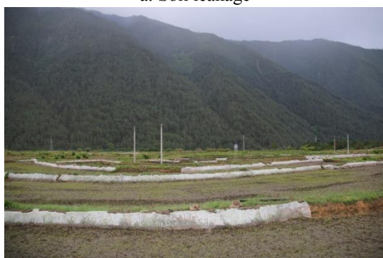
c. Plastic film wrapped soil to prevent collapse
