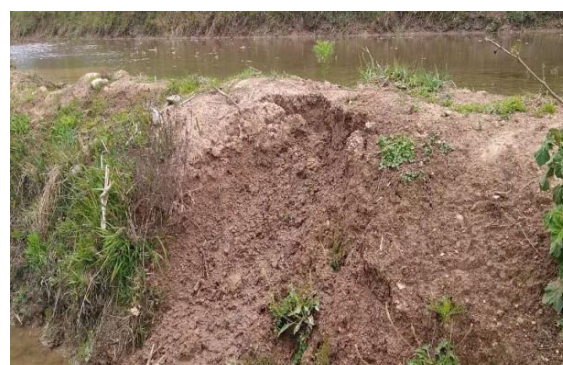
b. Soil collapse
