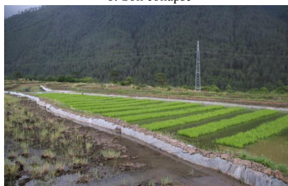
d. Plastic wrap around the soil to prevent water leakage
