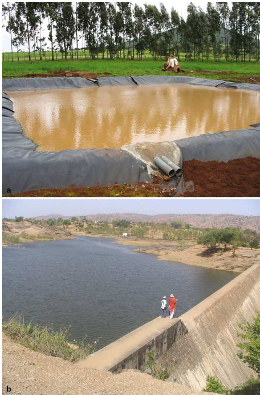
Fig. 28.2 a Water harvesting pond in the Nile basin with inflow and outflow structures. b Runoff collection pond in India with overflow weir
